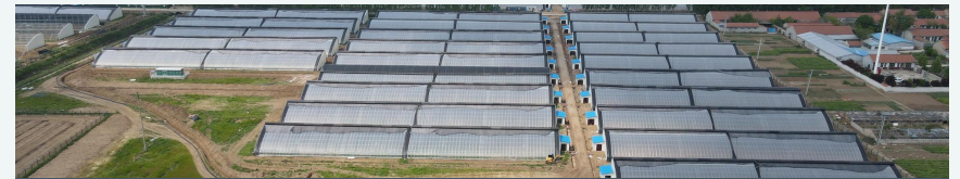
Greenhouse infrastructure | Shandong Lynwo
